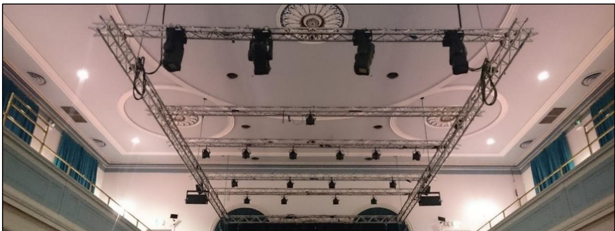
View of truss in raised position.
