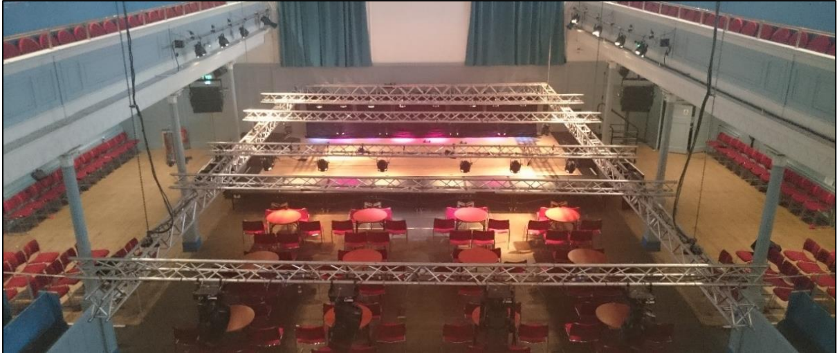
View of truss in lowered position.
