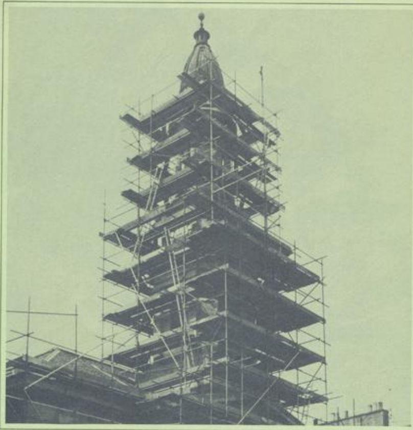
Below. Scaffolding round the belfry during stone-cleaning and repair work.
